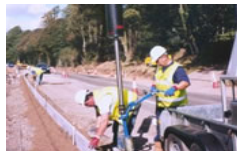
Laying a long run of kerbs with a vacuum lifter - an example of good practice
