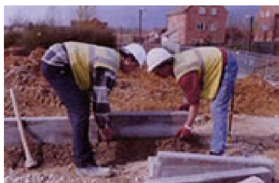
Laying a long run of kerbs with a vacuum lifter - an example of good practice
